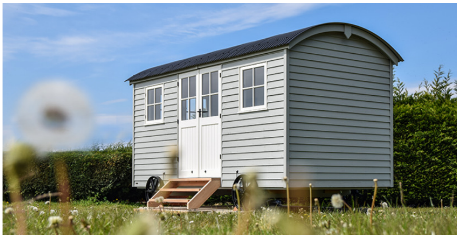
A small number of shepherd's huts such as this locally sourced product by Crane Garden Buildings, Narford, Norfolk to be scattered among the trees in the woodland.
